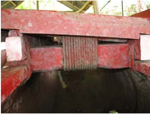
Figure 4a: Lashing of transverse beams to outrigger booms.
