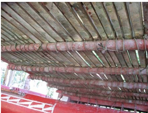
Figure 6a: Under the deck: lateral braces
